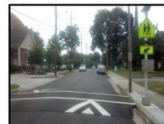
**Raised Intersection:** Raised intersections are flat raised areas covering an entire intersection with ramps on all roadway approaches. These devices are the same elevation the sidewalk, or slightly below to provide a “lip” that is detectable by the visually impaired. By modifying the level of the intersection, the crosswalks are more readily perceived by motorists to be “pedestrian territory”.
