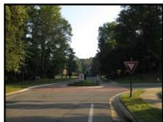
**Mini-Roundabout:** A Mini-roundabout consists of a circular raised island located in the middle of an intersection around which traffic circulates. These devices provide traffic calming benefits to neighborhood intersections by reducing speeds and crash severity.
