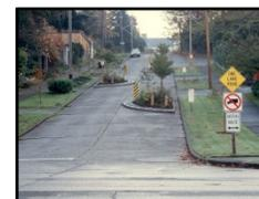
**Chokers:** Chokers are curb extensions at midblock locations that narrow a street by widening the sidewalk or planting strip. Two-lane chokers leave the street cross section with two lanes that are narrower than the normal cross section. One-lane chokers narrow the width to allow travel in only one direction at a time, operating similarly to one-lane bridges. They are good for areas with substantial speed problems and no on-street parking shortage.
